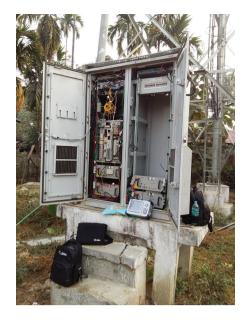
CellAdvisor tapping the BBU-RRH CPRI link — all measurements are at ground level
