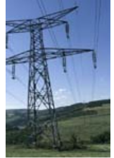
Figure 3: Picture of an OPGW
