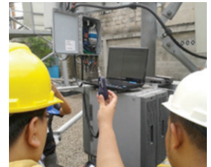
At the RRU (tower structure or rooftop)
